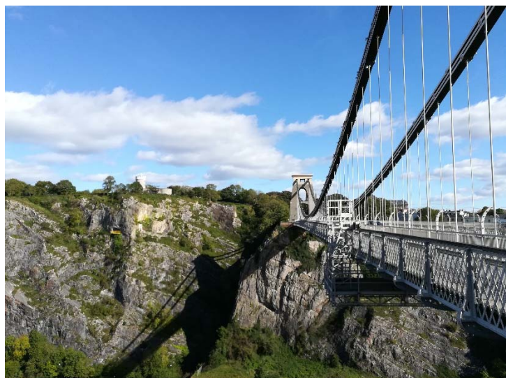
Clifton Suspension Bridge
